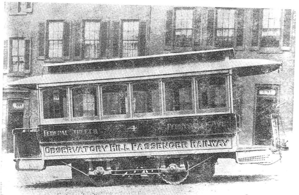
WHEN THE century was young, Number 4 mountaingoated up steep Federal Street and Perrysville Avenue. Power came from conduit
